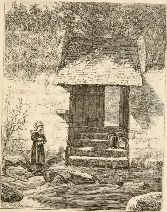
Washing-Place on the River.
